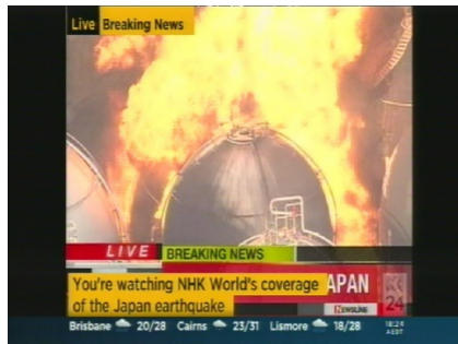
Fire at Onagawa Nuclear Power Plant, caused by Mw9.1 Tohoku earthquake
